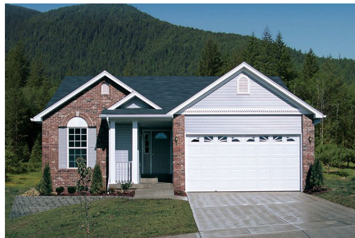
Garage and driveway are too prominent. Porch and columns are not balanced with other massing. Material shifts are forced.
