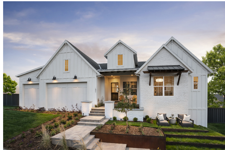
This modern farmhouse has balanced massing with a featured entrance and simple gable elements complemented by split pitches and metal awning roof details.
