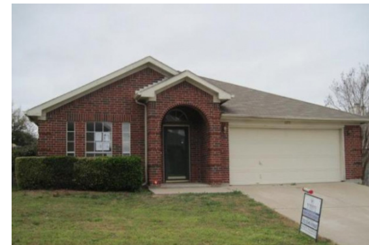
Paired windows are detailed improperly. The garage is too prominent in the elevation.
