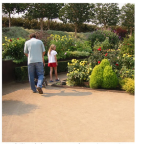
Stabilized decomposed granite paving
