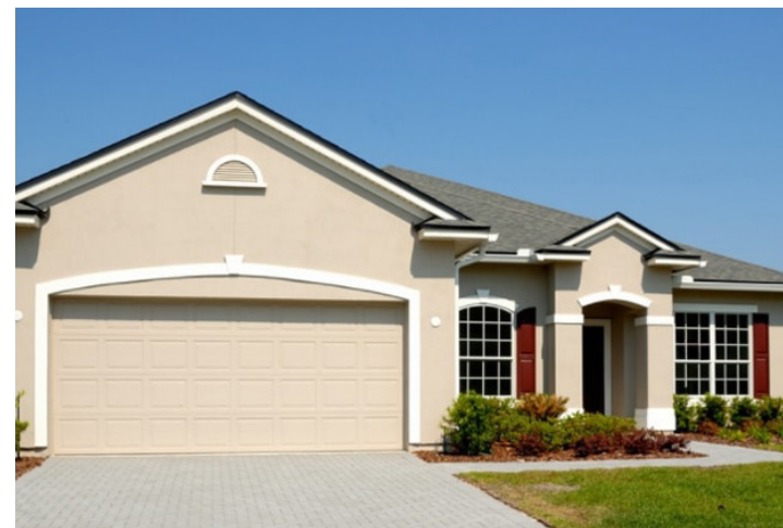
Elevation lacks symmetry and has no clearly defined style. Shutters are inappropriately sized for window openings.
